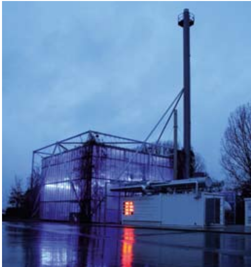
Co-generator powered by renewable raw materials
